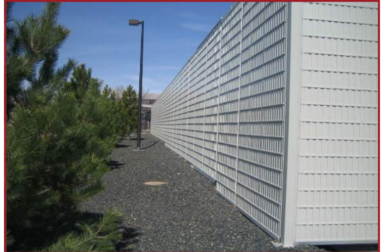
LSE Ground-level Enclosure
